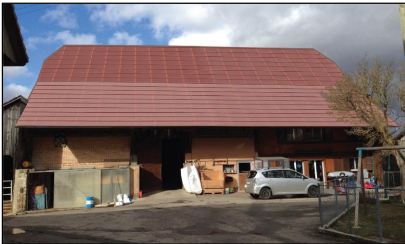
Slika 21: Pilotni projekt v Ecuwillensu, kanton Fribourg (Švica) z vgradnjo modula "Solar-Terra". (Vir: http://www.issol.eu/wp-content/uploads/2017/07/Brochure-227x190-SolarTerra-FR-4mb_2.pdf , 2020).
